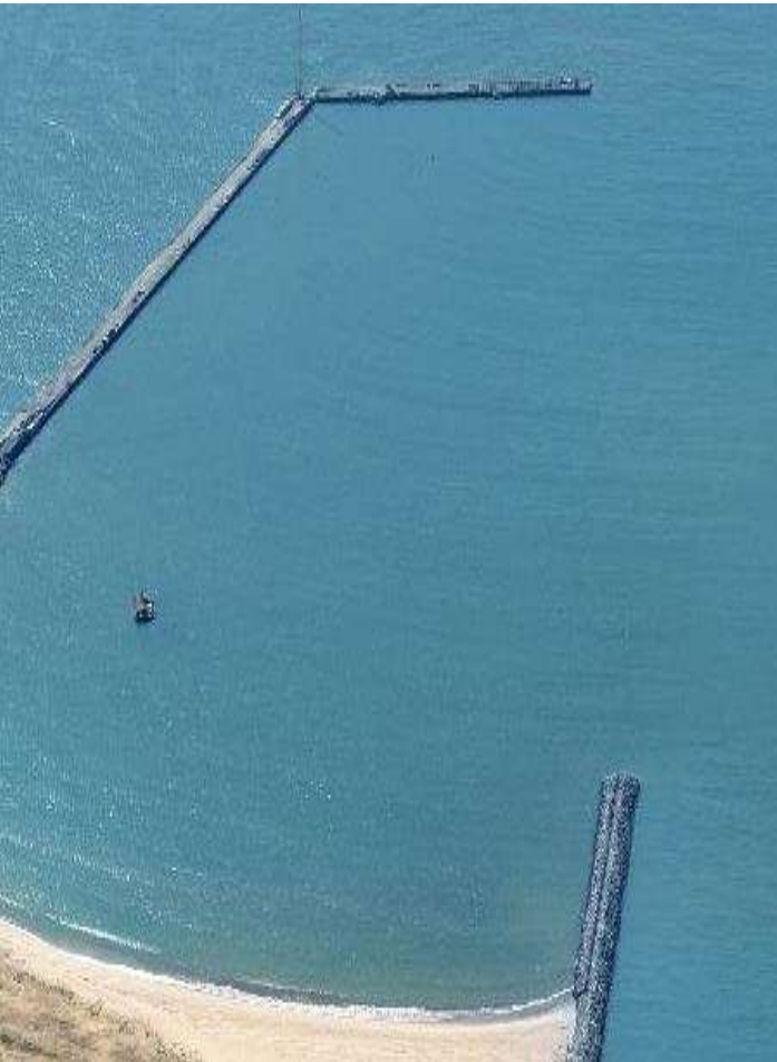
Caissons used for breakwaters
