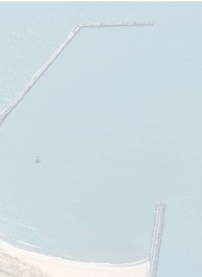
Caissons used for breakwaters
